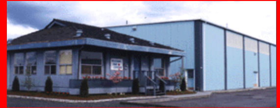
WFCi's Office and Laboratory at 2204 Parrott Way in Kelso, Washington.
